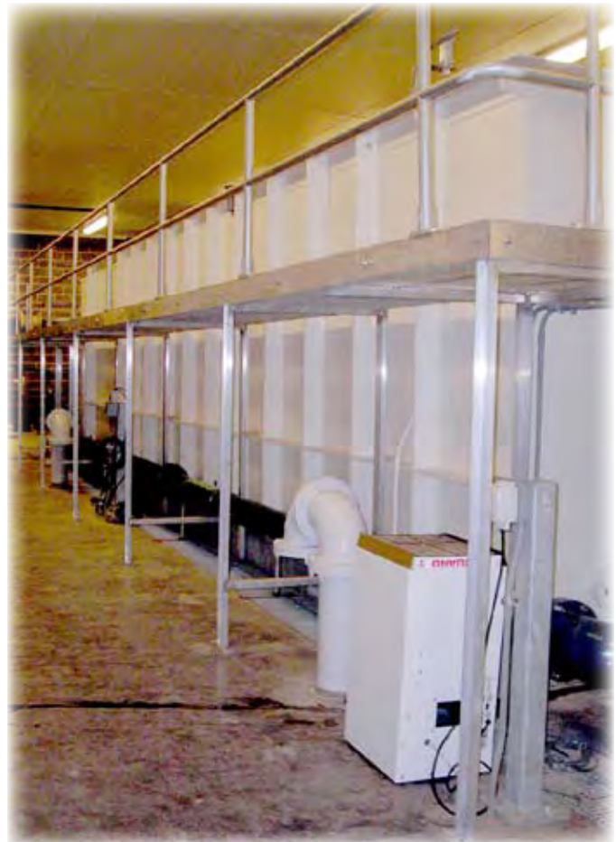
Pre-fabricated iron and manganese filter units in the main treatment room
